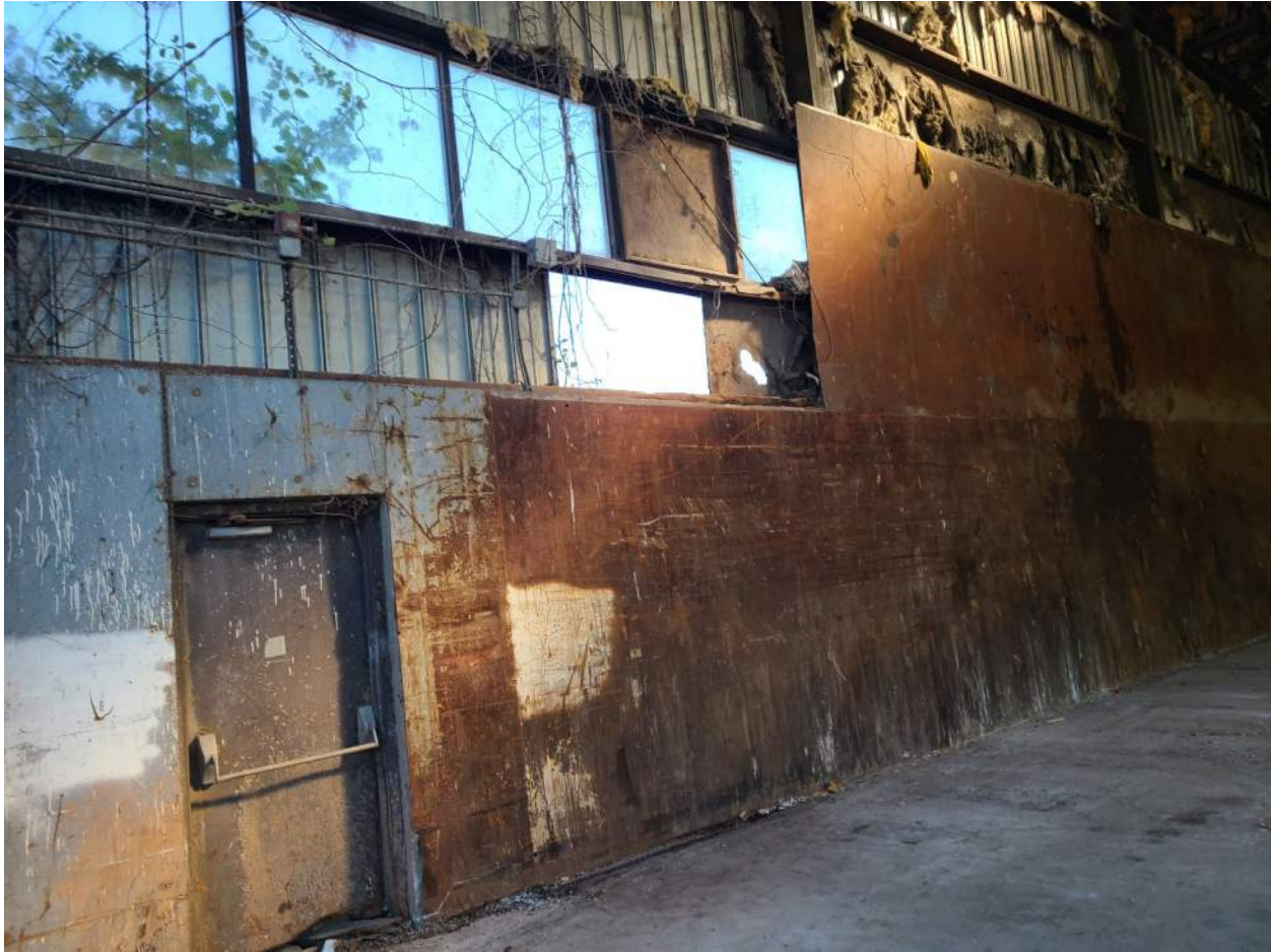
Interior View – Broken Wall Panels and Insulation
