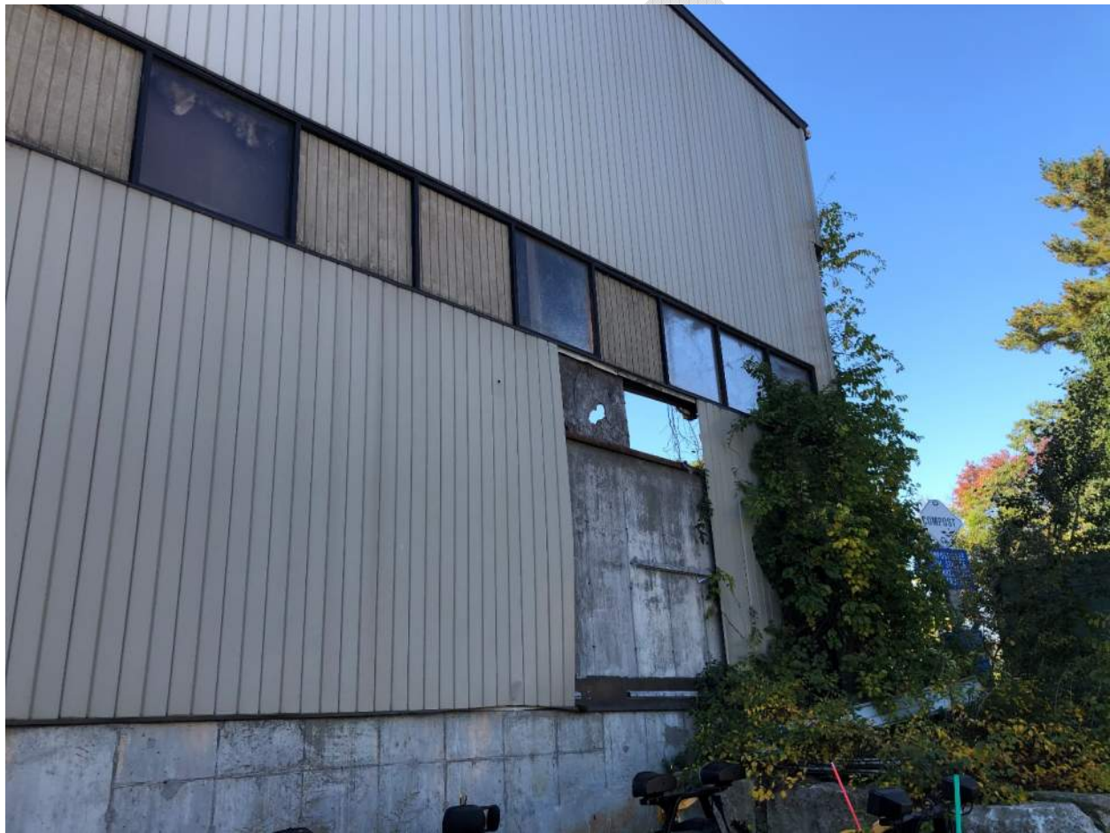
Exterior View - Broken Wall Panels
