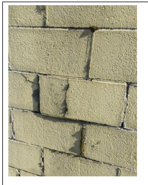
South Wall Impact Damage
