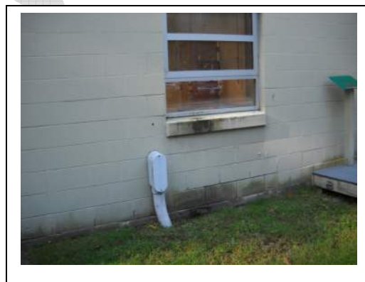
North Wall Water Infiltration at Grade
