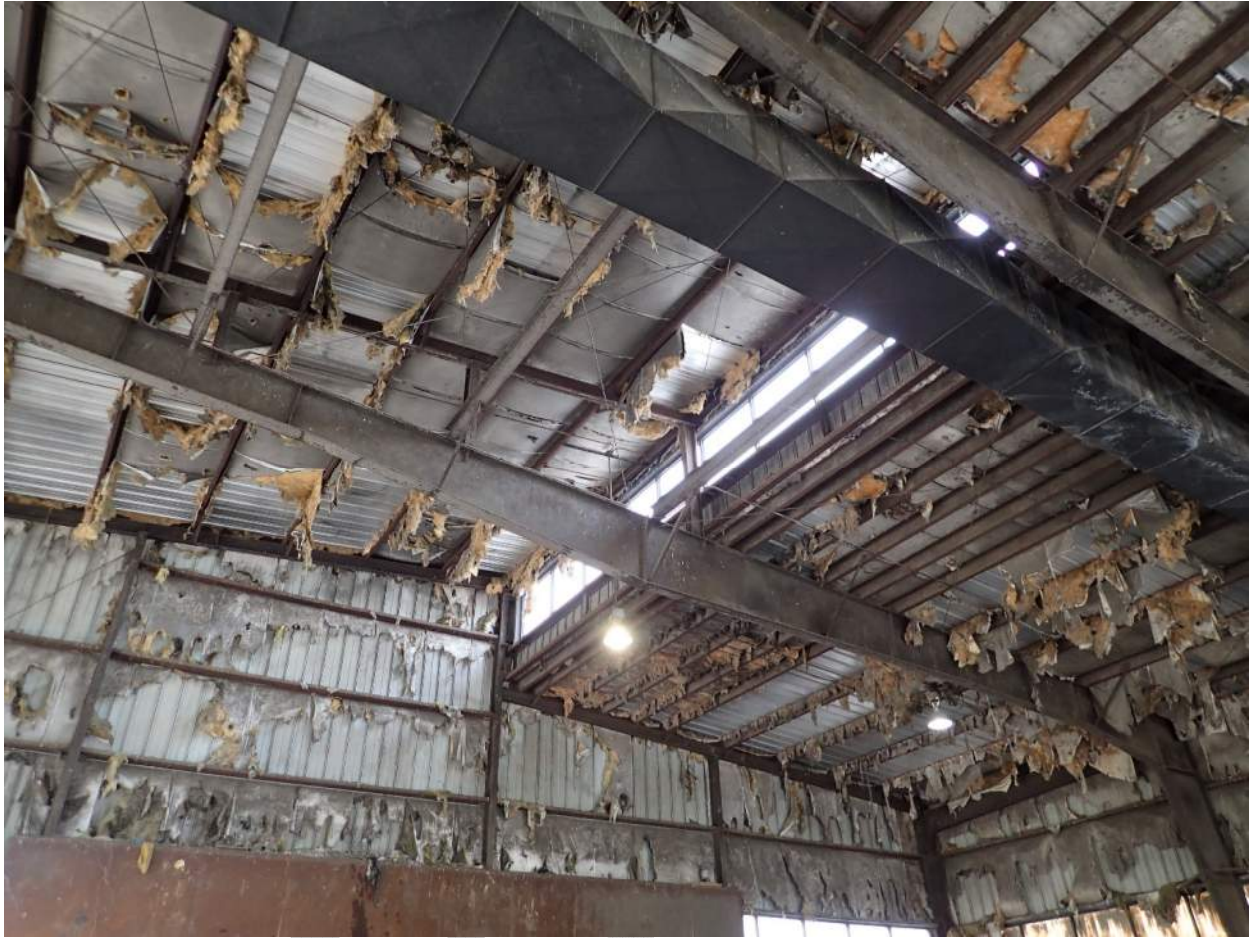
Interior View – Rusty Rigid Frame and Purlins
