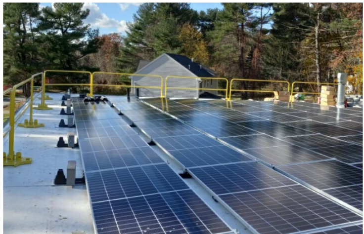
Solar panel installation on the roof of the new North Acton Fire Station on Harris Street. Consistent with net zero goals, this building utilizes geothermal ground source heat pumps and is not connected to natural gas.
