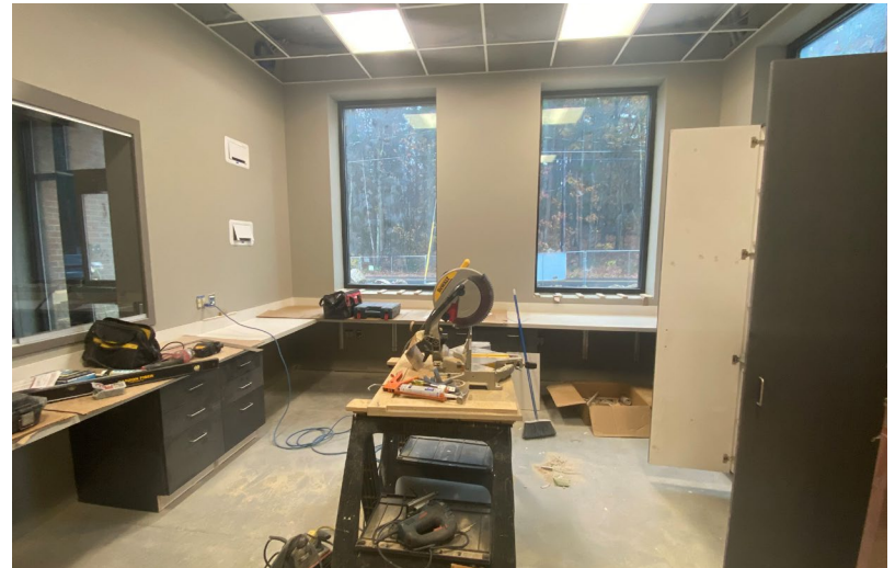
Millwork installation
