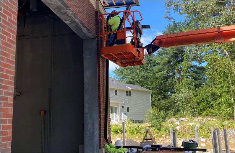
Installation of gutter on north side of the building
