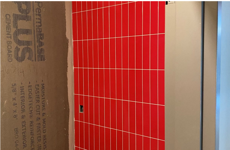
Grouting the tile in the bathroom wall
