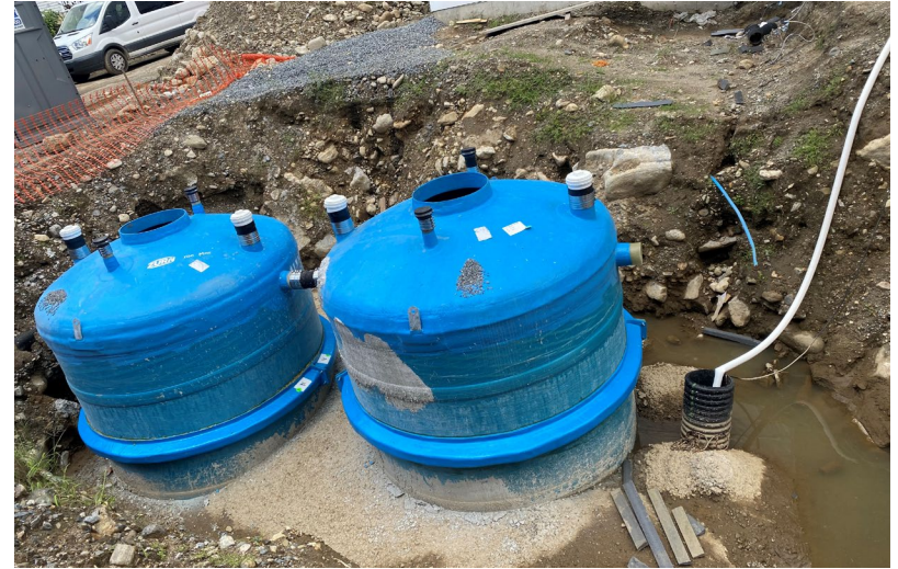
GSI tank reinforcement install
