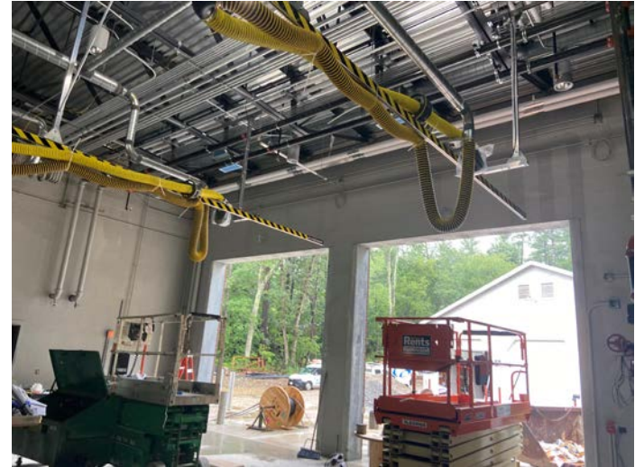
Painting of apparatus bay walls on north side
