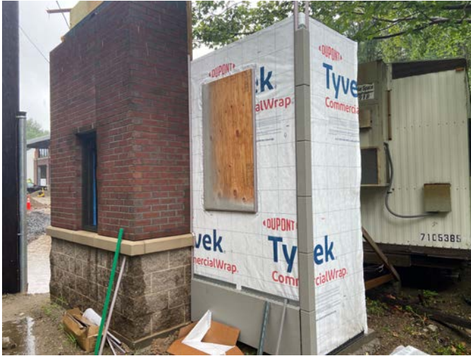
Installation of Nichiha panels on mockup
