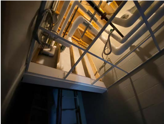
Acoustical ceiling grid installed in storage room
