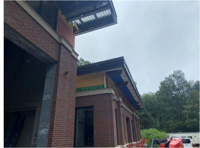
Installation of vapor retarder at soffit
