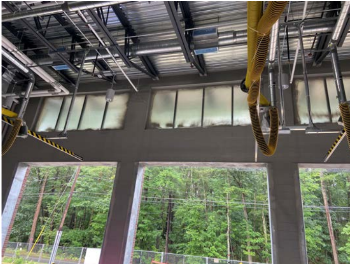
Painting of apparatus bay walls
