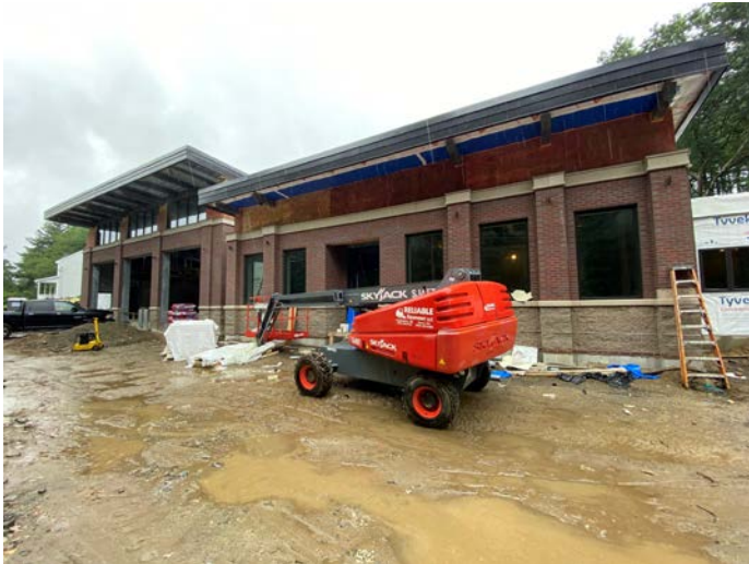
Overview of southeast side of building
