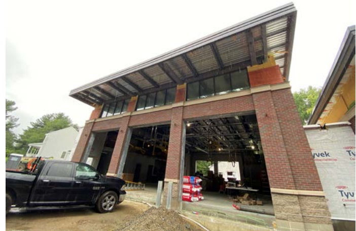
Overview of apparatus bay from south side
