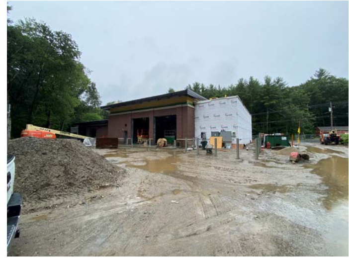
Overview of north side of building
