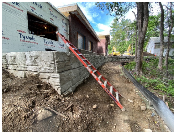
Retaining wall installed (05/28/2021)
