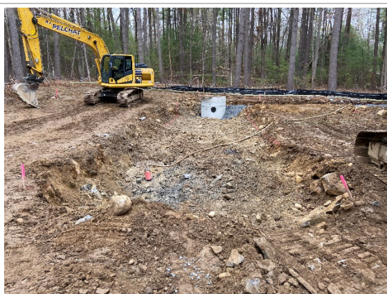
Overview of excavation for infiltration system #1 (04/29/2021)
