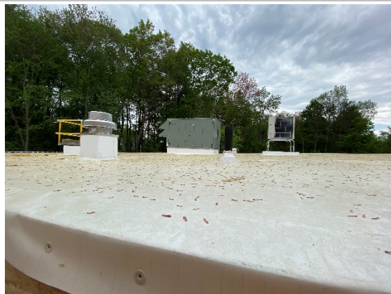
Rooftop units installed on east side. Connections to be made to units. (05/21/2021)
