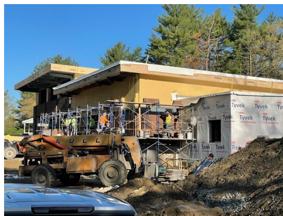
Installation of masonry façade on south side (05/07/2021)
