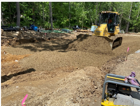
Pavement subgrade preparation on west side of existing garage (05/27/2021)
