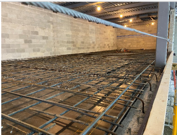
Western mezzanine slab reinforcing installation (04/15/2021)
