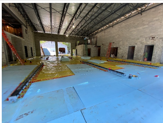
Vapor barrier and rigid insulation installation of apparatus bay (05/19/2021)
