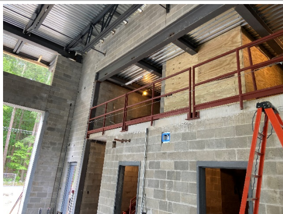
Installation of mezzanine railing (05/28/2021)
