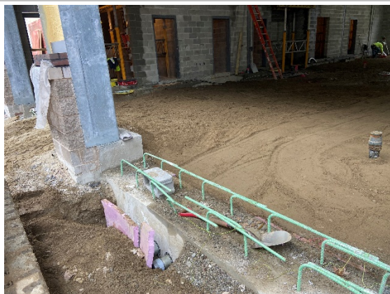
Realigned electrical conduits for emergency power and telecom lines and compacted graded apparatus bay subgrade (04/29/2021)
