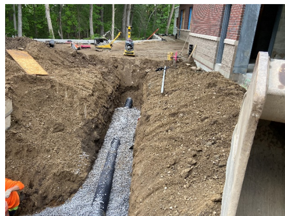
Installation of area and roof drains on north side (05/28/2021)
