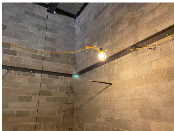
Mezzanine slab edge supports installed (04/13/2021)
