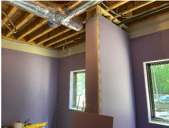
Start of below ceiling drywall in bunk areas (05/27/2021)
