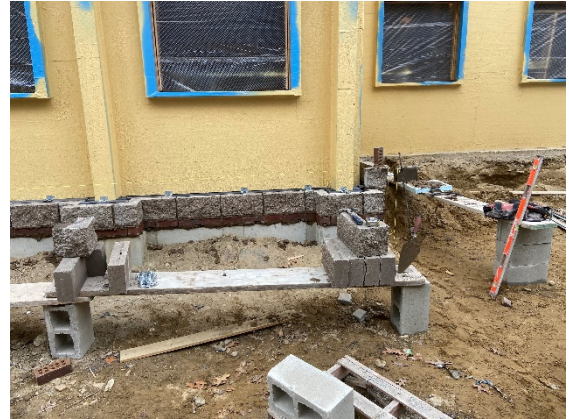
Masonry façade construction on south face (04/15/2021)
