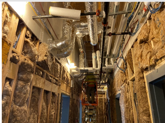
Installation of MEP pipe and duct insulation on east side (05/17/2021)
