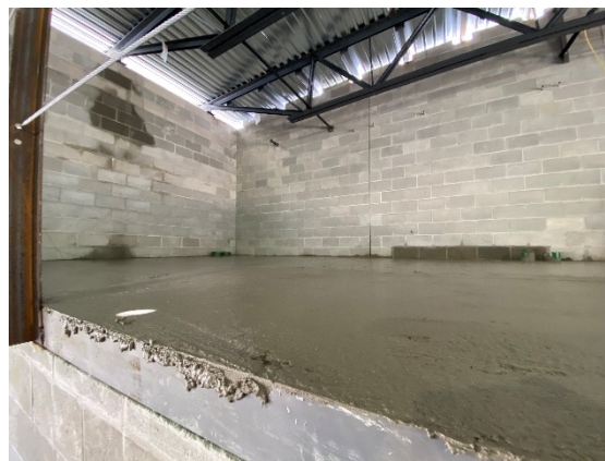
Concrete placed at dirty laundry room roof (04/20/2021)
