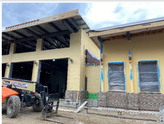
Masonry façade on south face and transition roof (04/21/2021)
