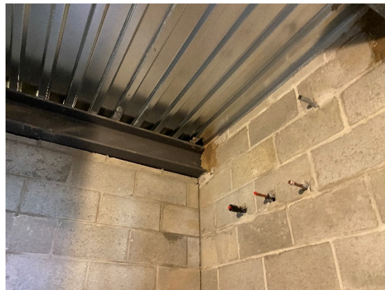
Typical grouted beam pockets at CMU wall (04/23/2021)
