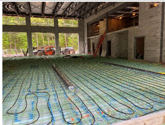
Installation of apparatus bay radiant heating and slab reinforcement (05/21/2021)
