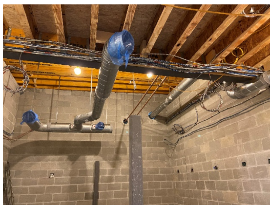
MEP rough-ins in gear room (04/13/2021)
