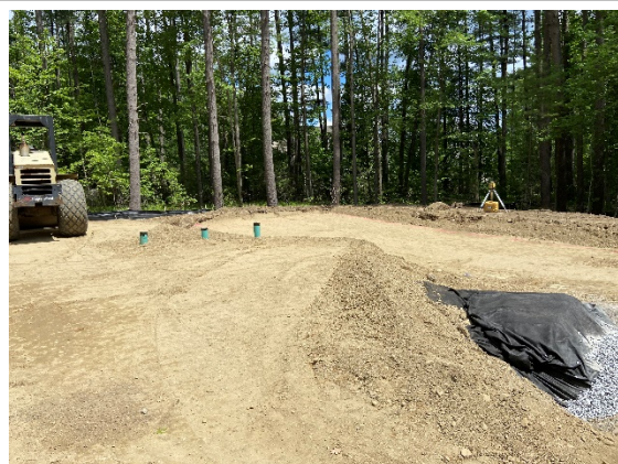
Backfilled stormwater infiltration system 1 (05/24/2021)
