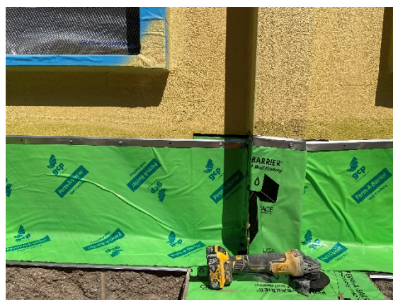
Typical drip edge and raft installed at south face (04/20/2021)
