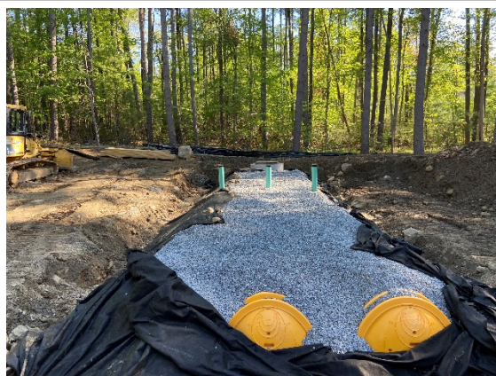
Installation of stormwater infiltration system 1 (05/17/2021)
