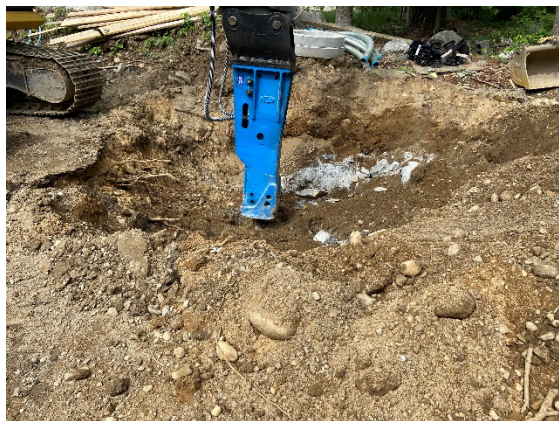
Removal of rock mass at CB 2 (05/28/2021)
