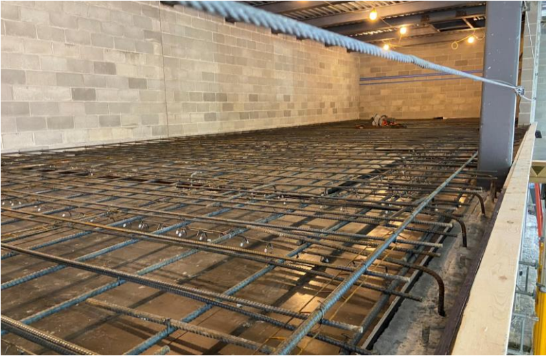
Reinforcing installation for mezzanine slab
