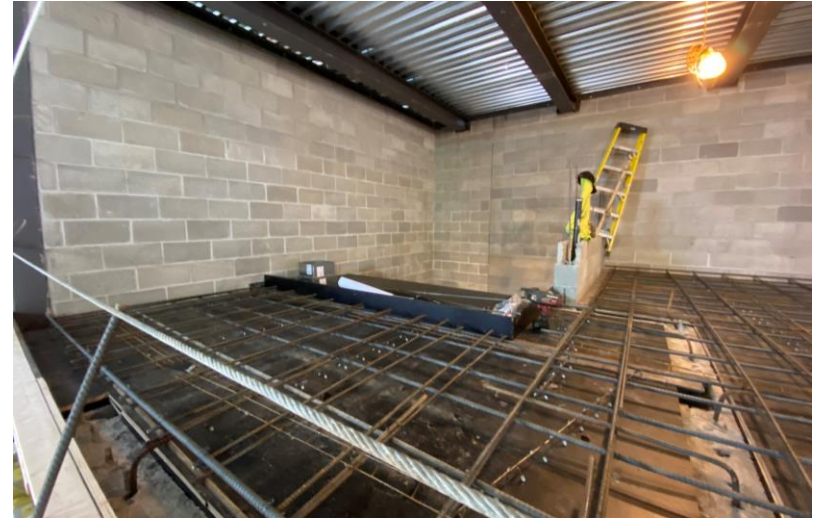
Reinforcing installation for mezzanine slab looking towards south stairs
