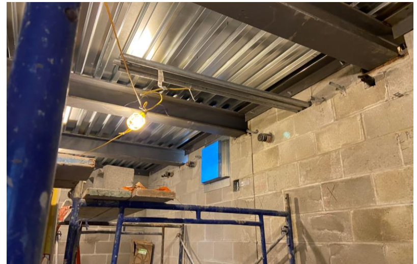
Metal deck roof installed at dirty laundry room
