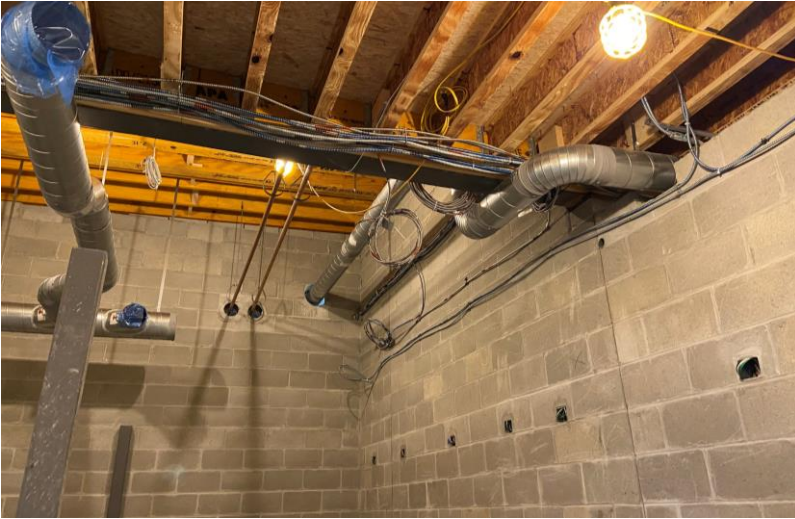
MEP rough-ins at gear room
