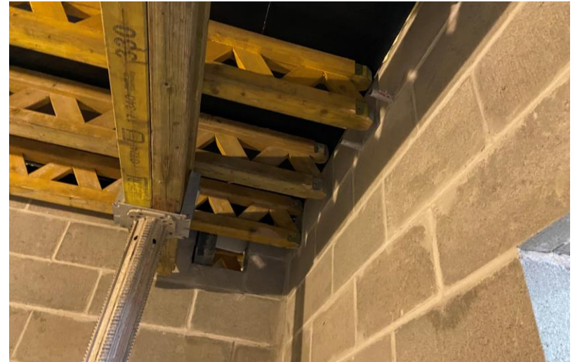
Typical shoring underside for mezzanine slab
