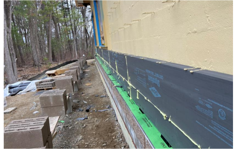
Flashing installed on north side
