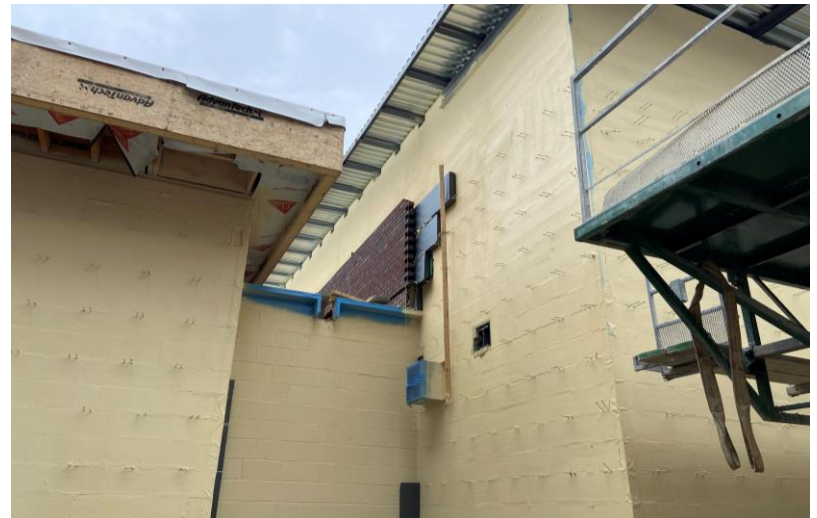
Façade installation at transitional low roof
