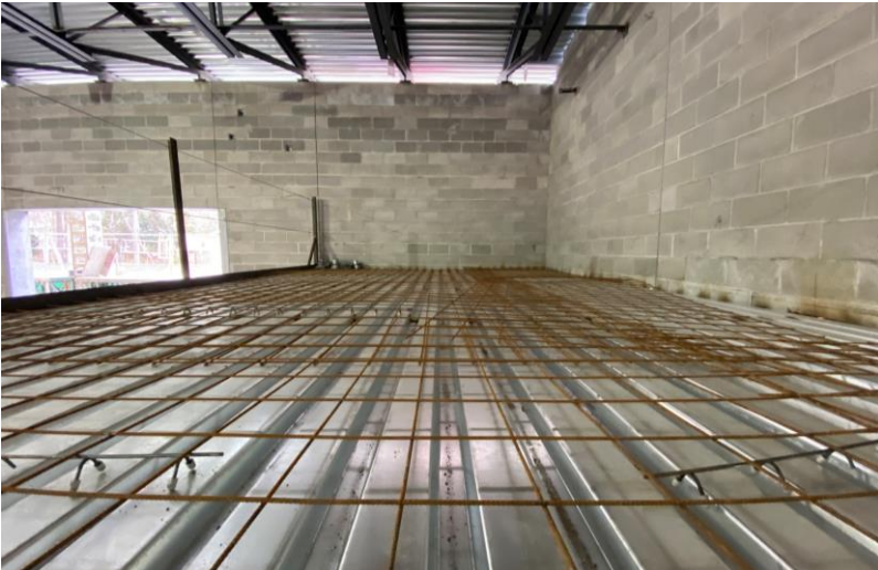
Reinforcing installation for dirty laundry roof
