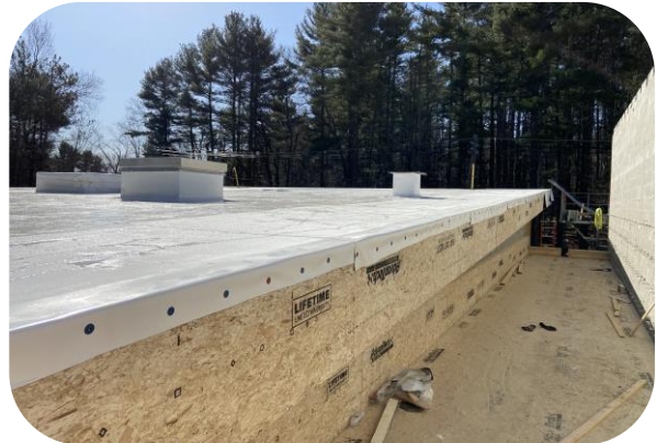
Roof hatch installed on admin side sloped roof. Roofing installed (03.23.2021)
