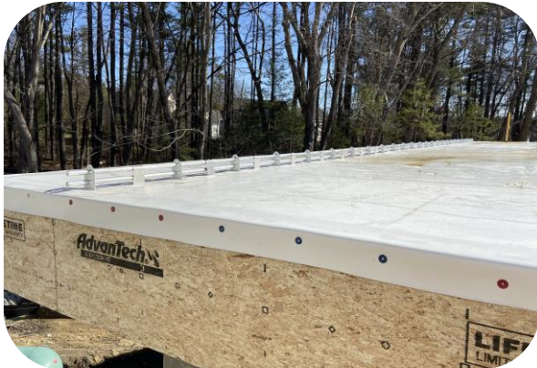
Snow fence on admin side sloped roof. Roofing installed (03.23.2021)
