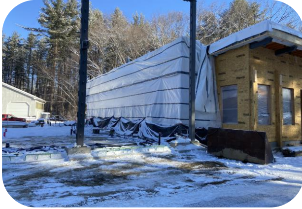
Overview of enclosed masonry scaffolding on west side of wood construction
