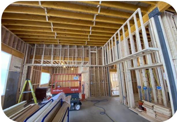
Interior soffits and wood wall framing
