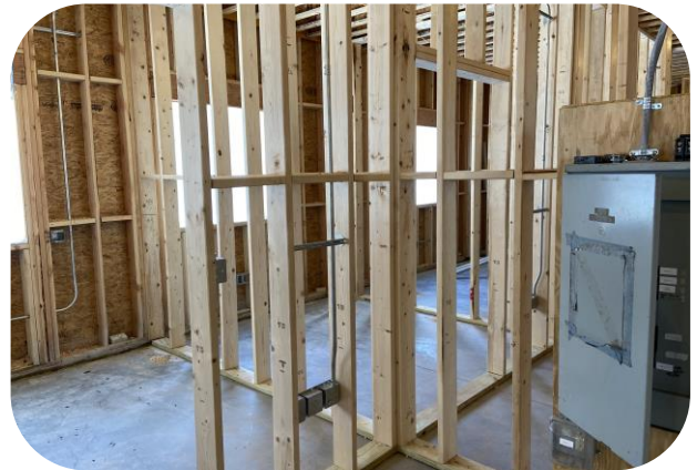
Electrical rough in
