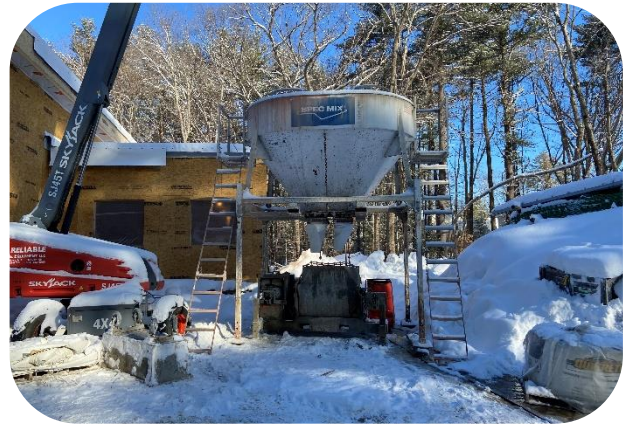
Grout plant set up
