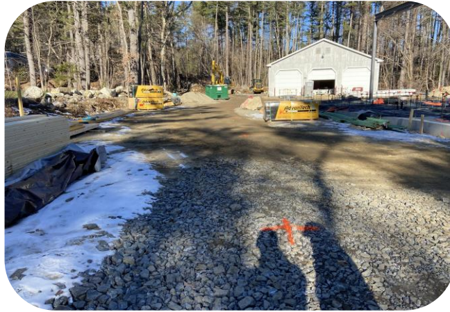
Markouts for geothermal wells
