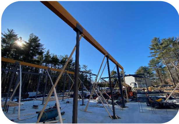
LVL joists installed on east side of building
