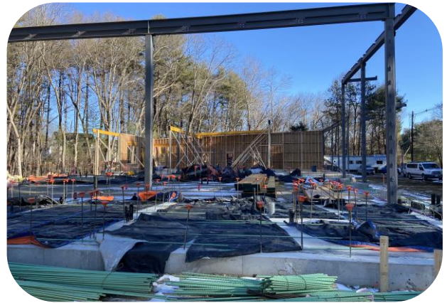
Overview of wood construction from southwest side
