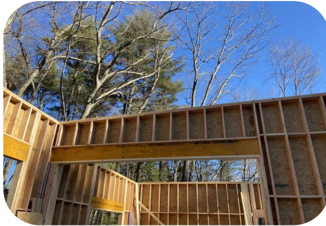
Interior wood construction on east side of building
