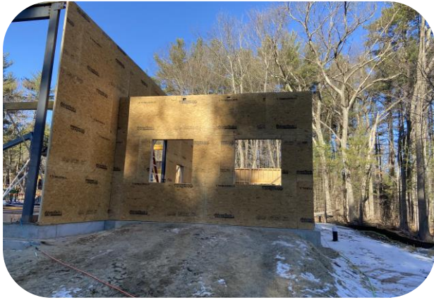
Interior and exterior wood construction on east side of building
