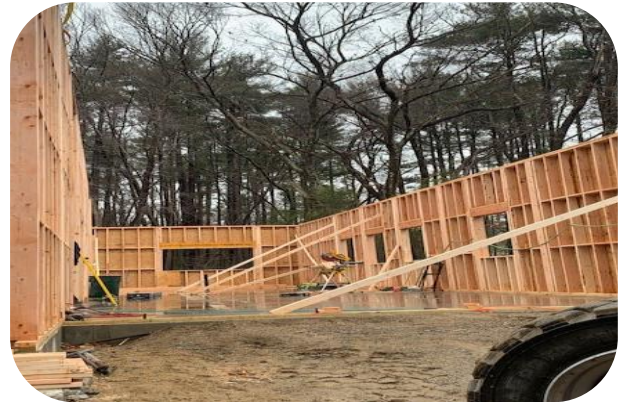
Interior and exterior wood framing construction on east side of building
