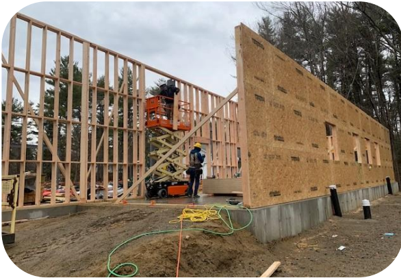
Interior and exterior wood framing construction on east side of building
