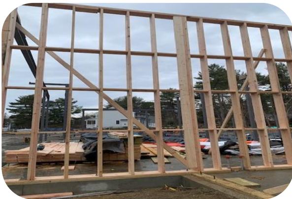
Interior and exterior wood framing construction on east side of building
