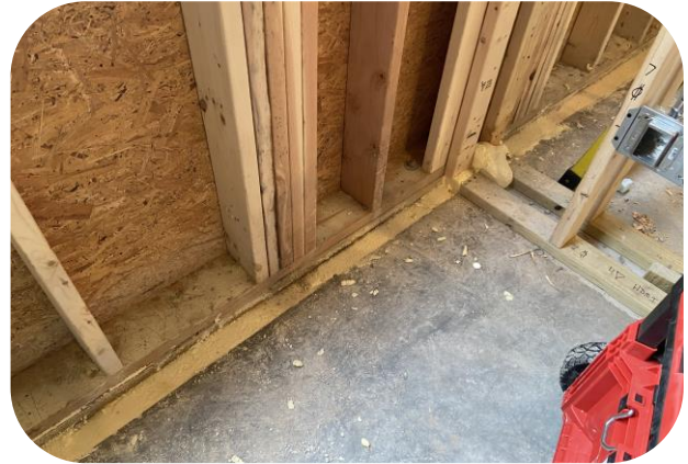
Slab edge insulation installed on east side
