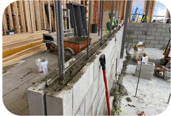
Installation of bond beam
