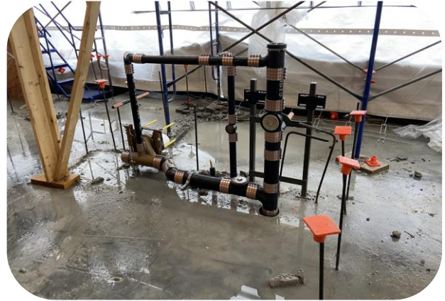
Plumbing rough-in and removal of lightweight CMU blocks (02/16/2021)
