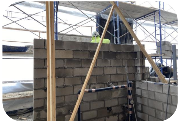
Masonry installation and plumbing rough-in
