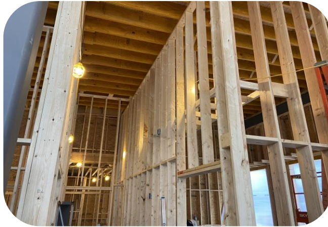
Interior soffit installation in conference room on east side
